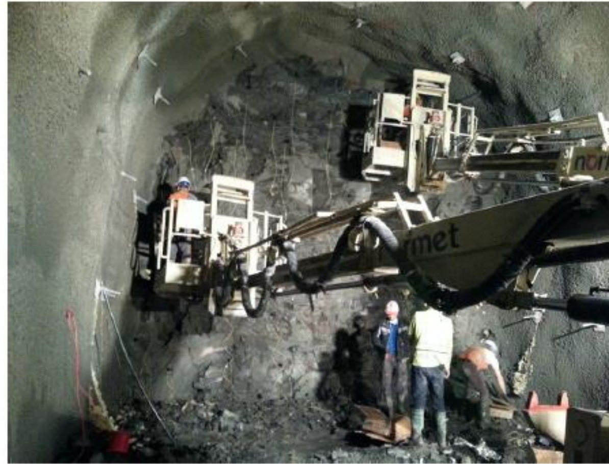
Preparation for Explosion (Drilling) in SAT1
