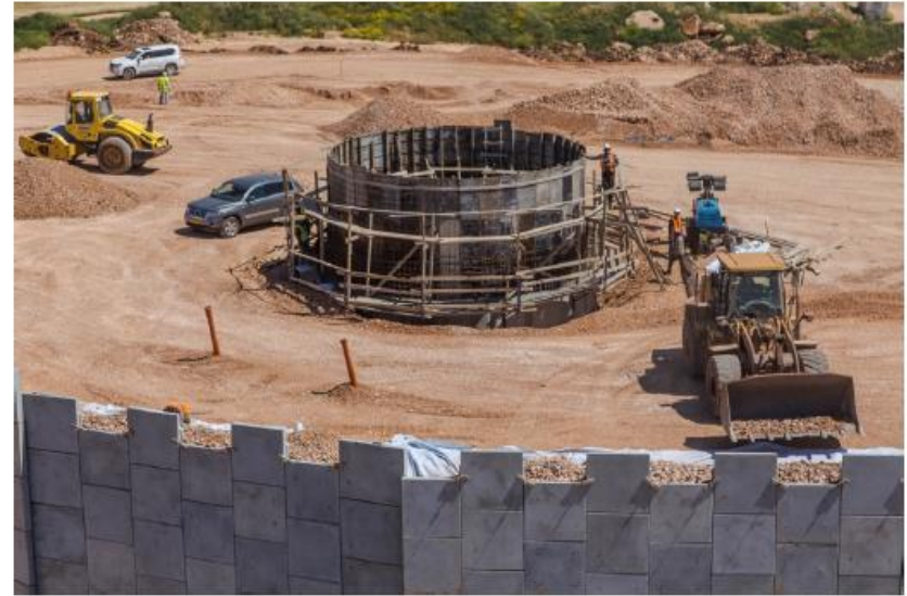
Upper Reservoir Cylinder Completion Concrete Works
