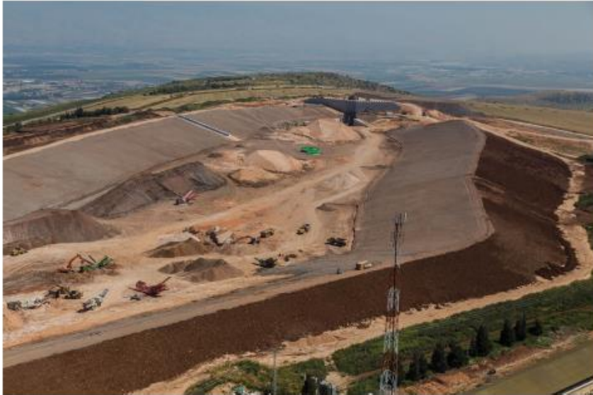
Upper Reservoir Embankment Works
