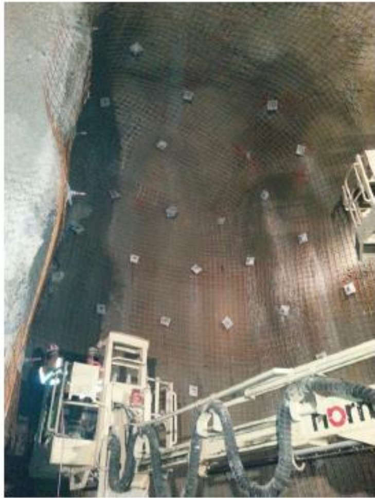
Execution in Power House Cavern
