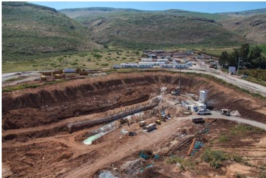
Lower Reservoir Intake Foundation Works
